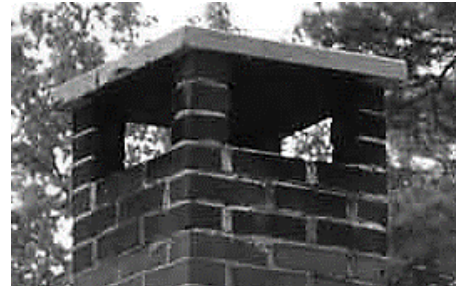
Concrete Cap Chimney Top
