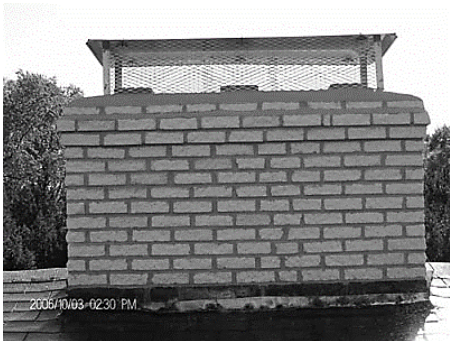
Metal Cap on Clay Liner Chimney Top
