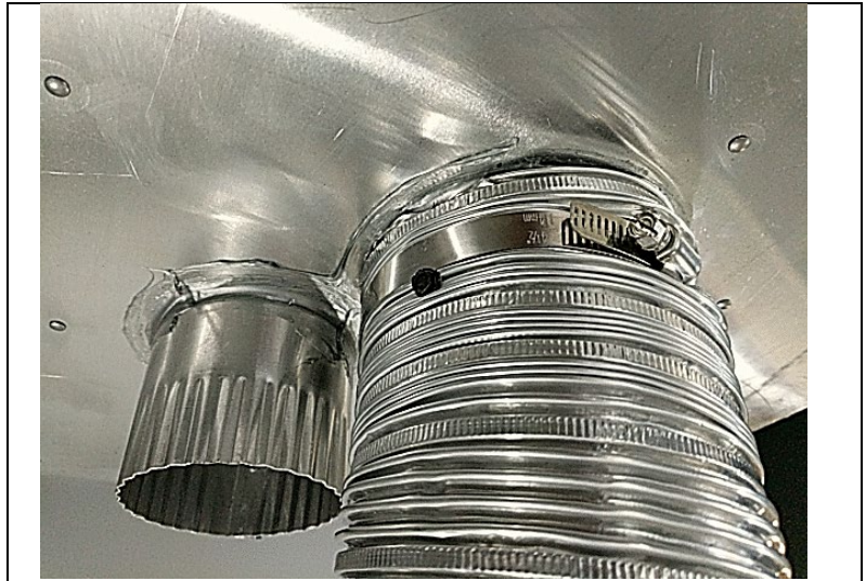
Hose Clamp first. Secure w/ Screw above Hose Clamp
